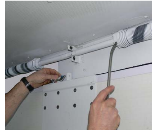
Figure 1 – Adjusting the door balancer
